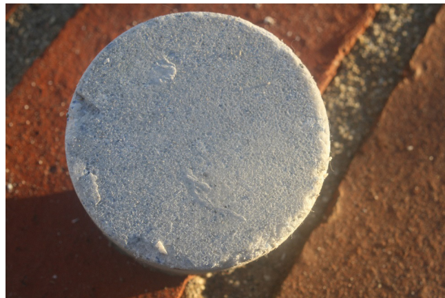
Figure oB-00045 – Front of Core with Craze Nodules Following Cracks
