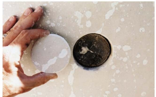
Figure oB-00015b – Front of Core with Crack and Nodule Following Crack
